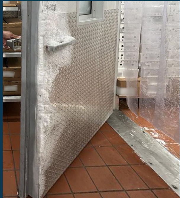
Left, a Medium-security Facility Refrigerator Door Not Fully Sealed, Right, Ice Accumulation on the Door of a Medium-security Facility Walk-in Freezer
