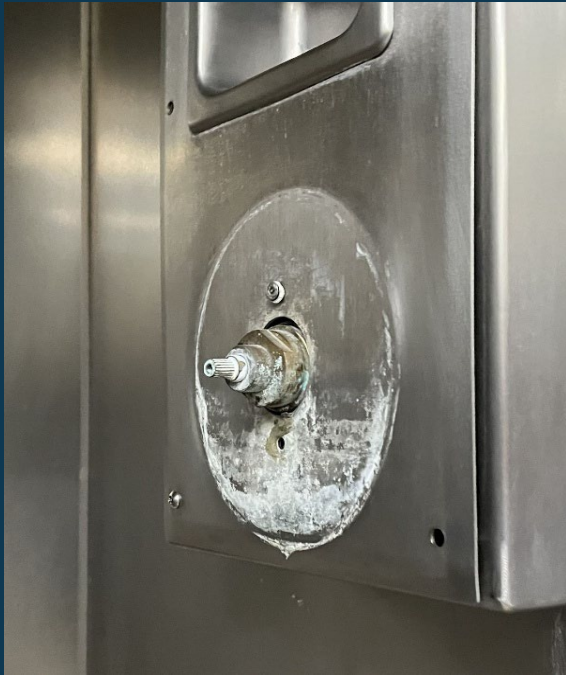
Left , a Shower with a Missing Handle at the Camp, Right , a Broken Showerhead at the Camp That Continuously Leaked Water
