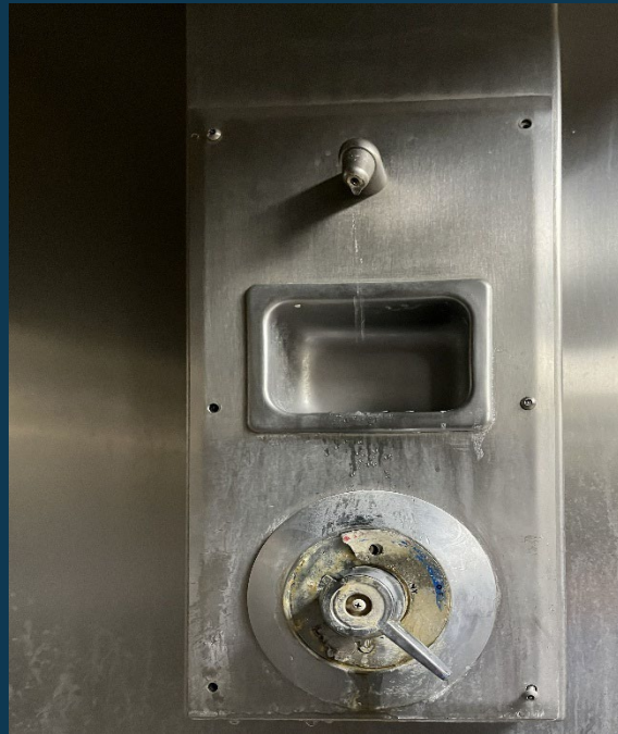
Left , a Shower with a Missing Handle at the Camp, Right , a Broken Showerhead at the Camp That Continuously Leaked Water
