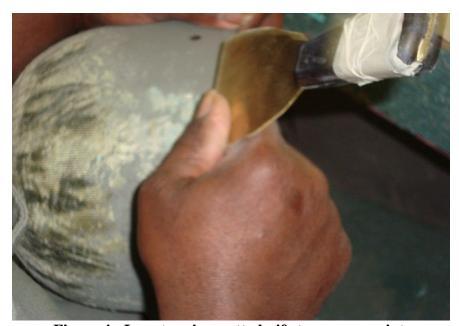
Figure 4: Inmate using putty knife to remove paint.
